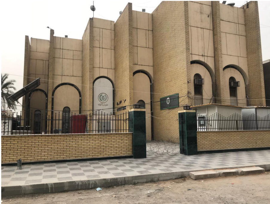
Figure 17 Al-Rafidain Bank building in Al-Mansour
