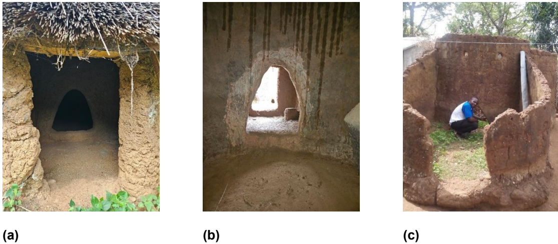
Figure 27: View of the Two (02) Access Openings to the Women's Hut
