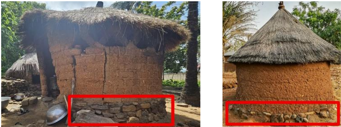
Figure 16: Photos Showing the Reinforcement of the Foundations by the Stones
