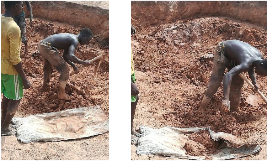
Figure 10: Stage Of Digging Up the Earth and Near a Construction Site.
