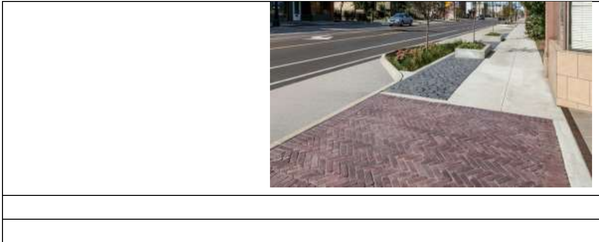
(Figure 6) Sidewalks and Pavements
