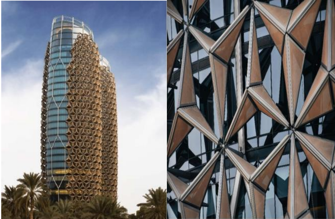
Figure 1: (: Al Bahr Towers – Abu Dhabi- Project 1) The interactive facade of the Al Bahr Towers building in Abu Dhabi, showing the dynamic facade system for controlling solar radiation. Image adapted from. Attia et al. (2019) and used under a Creative Commons Attribution-Non Commercial 4.0 International (CC BY-NC 4.0) license.
