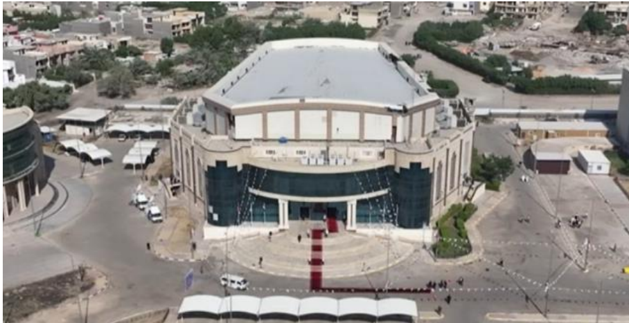
Figure 3: (Project 3) Sunni Endowment Building – Baghdad (P3): By the Media Office of the Prime Minister of Iraq - YouTube channel of the Media Office of the Prime Minister of Iraq, [1]. And https://ar.wikipedia.org/w/index.php?curid=9375661
