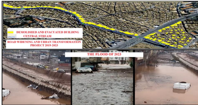
Fig. 13 Structures evacuated from the Karakoyun riverbed and the flood that occurred in 2023 (ŞBB 2025).
