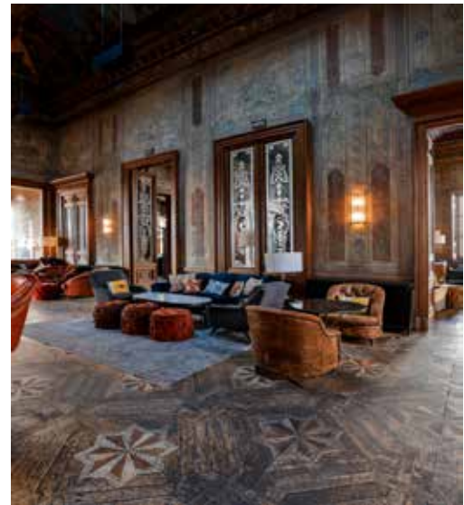
Fig. 12: Mahogany parquet flooring adorned with 8-point stars and herringbone patterns (URL 7, 8).
