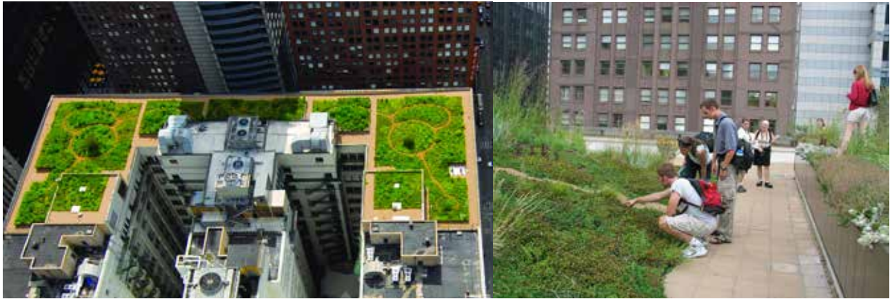
Figure 2. Green Roof City Hall. Source: TonyTheTiger, Chicago City Hall Green Roof. 2008, DigitalImage. Available from Wikipedia (URL- 2)
