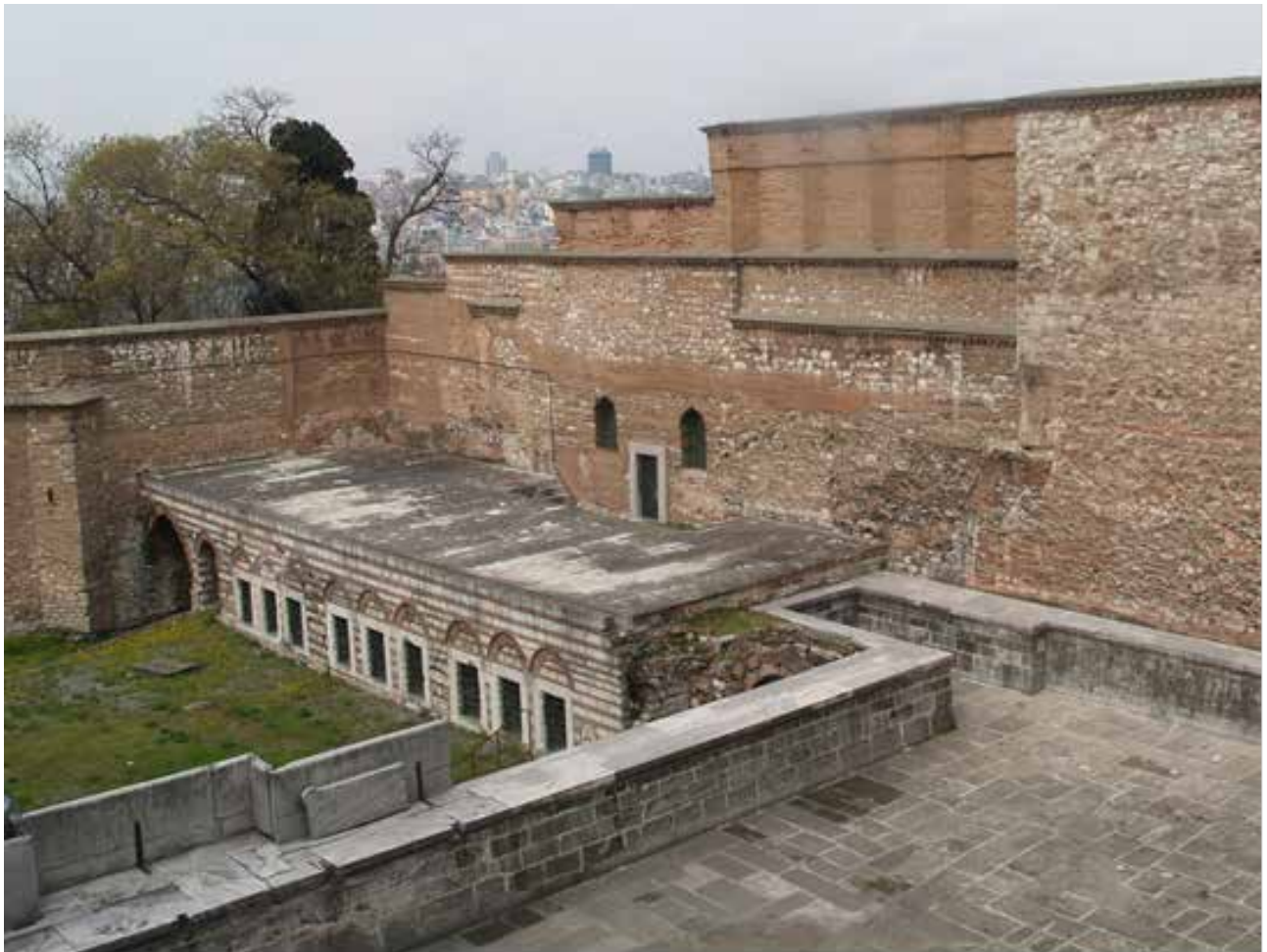
Fig.1 General View of Arslanhane-cage(Sedes Architects Archive)
