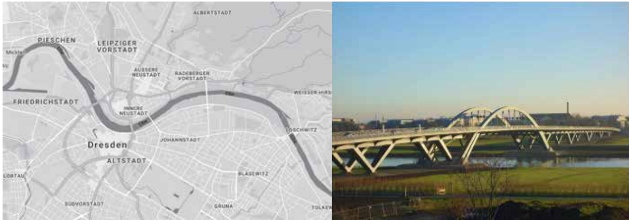
Figure 2: Dresden Elbe Valley Waldschlößchen Bridge construction location and image after the construction (Severinsen,A.L.B. 2020) (Asfa, 2019)
